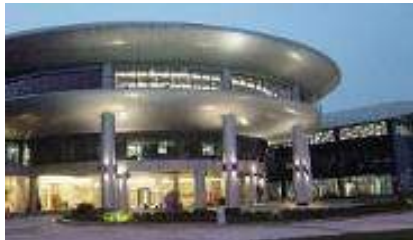
China Technology Center Shanghai, China
